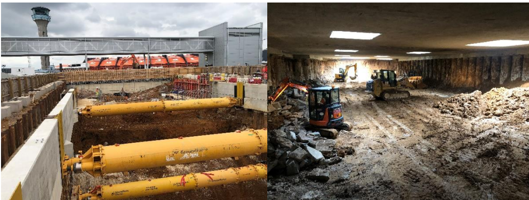
Inset 5.20: Open box and top-down construction on Luton DART scheme
