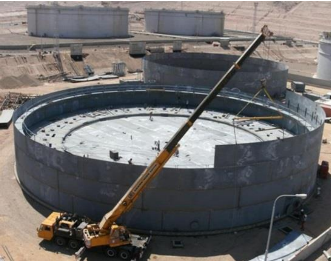
Inset 5.31: Example storage tank under construction (larger than the proposed)
