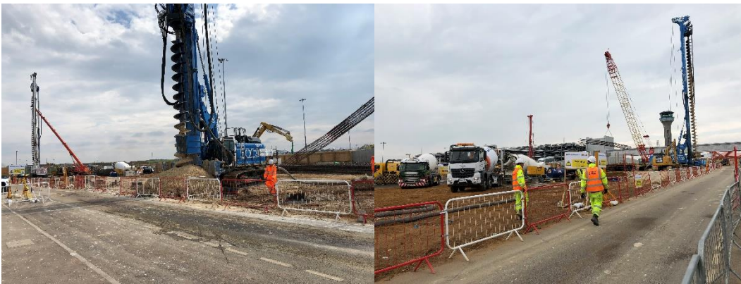
Inset 5.8: Typical CFA piling operations
