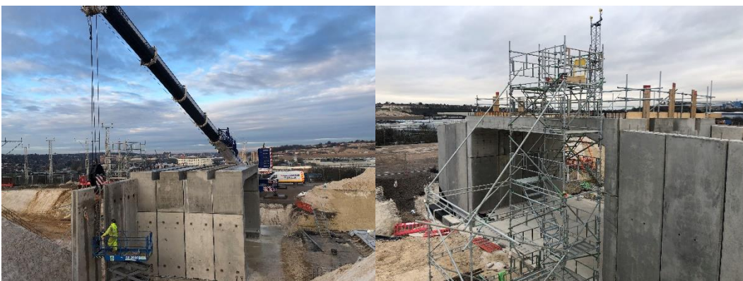
Inset 5.23: Precast sections on first Luton DART scheme
