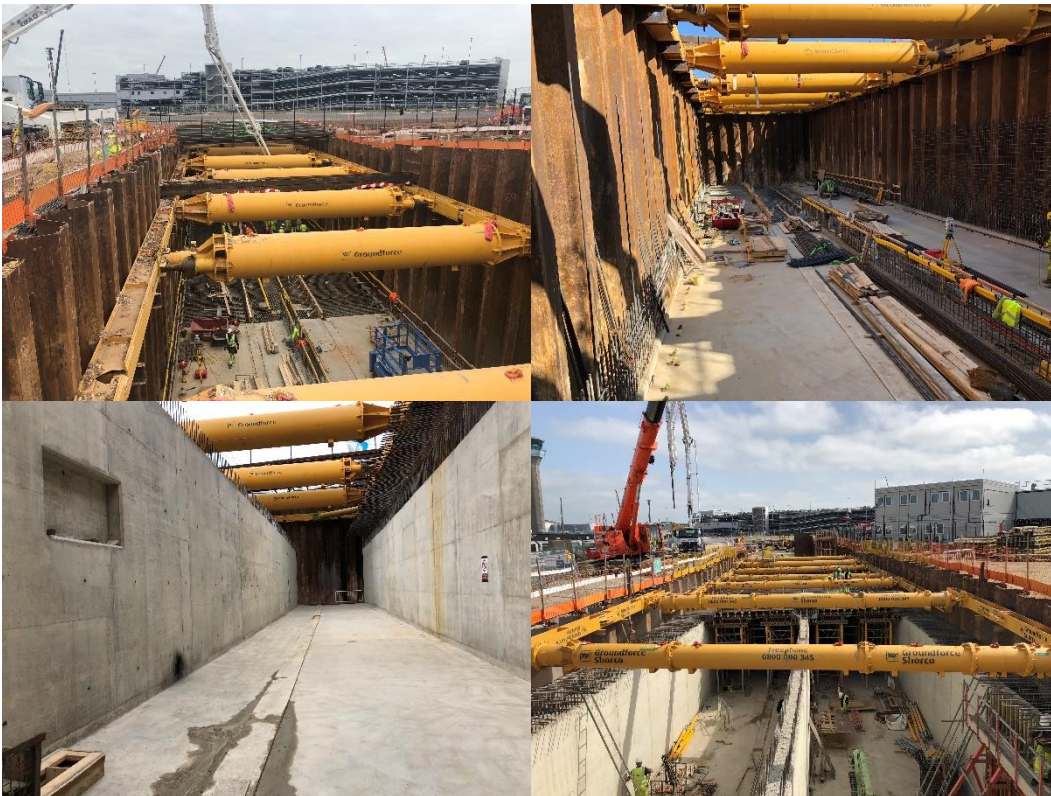
Inset 5.22: Sheet pile open box construction on first Luton DART scheme
